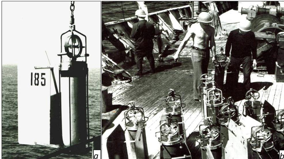
**Fig. 7.** MGI-1301 autonomous current and temperature meter designed in Special Design and Technological Bureau – *a*; complete supply of the Marine Hydrophysical Institute research vessels by the self-developed current meters – *b*
