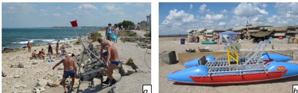
**Fig. 14.** Ways of “Donnaya Stantsiya” mounting: manually (the beach of Chersonesos Reserve) – *a*; by means of a specially designed watercraft on the basis of the inflatable catamaran “Neris” Tuzla Spit – *b*
