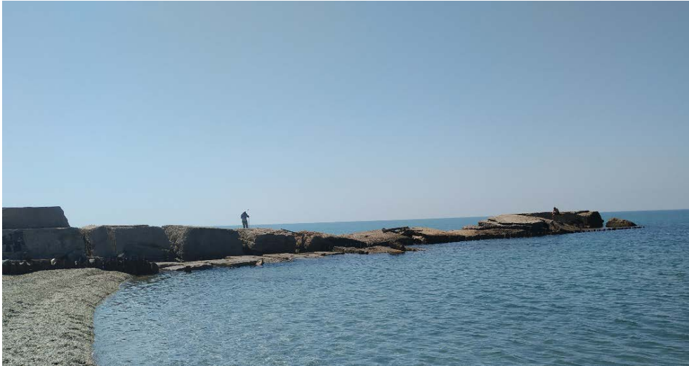
Fig. 3. Sea water intake on the Lake Sasyk bay-bar (view from the north)
