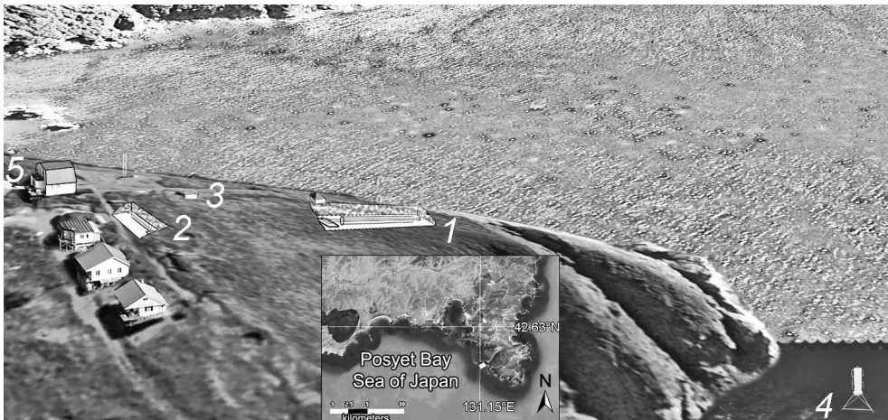
Fig. 2. Layout of laser interferometer locations: 1 – laser strainmeter with a measuring arm length 52.5 m; 2 – laser strainmeter with a measuring arm length 17.5 m; 3 – laser nanobarograph; 4 – laser meter of variations of hydrosphere pressure; 5 – laboratory
